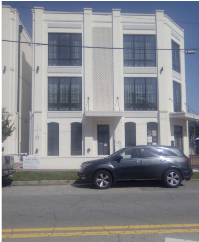
Front of Building
