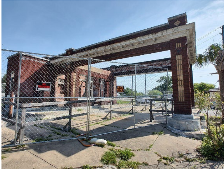
410 East 37 th Street Site Conditions in 2023
