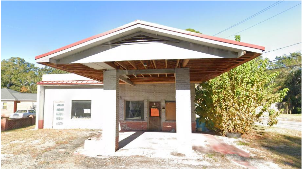
1028 Bonaventure Road – existing structure
