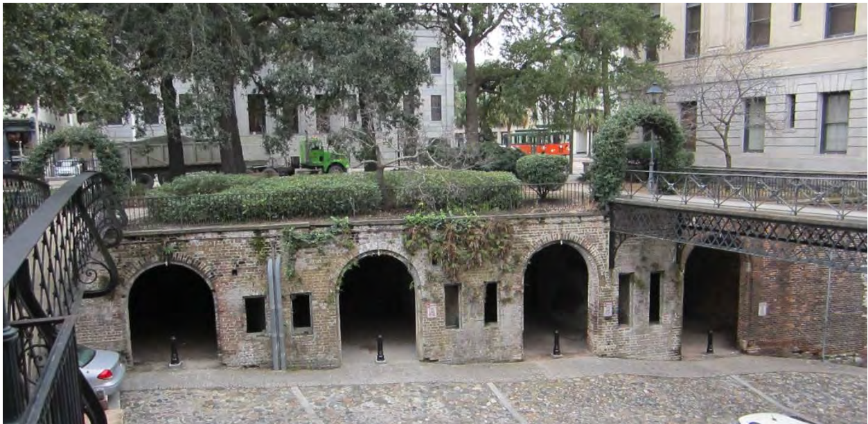
Looking south from the Thomas Gamble Building down at the Cluskey Vaults, City Hall is in the far right of the view.
