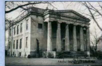
Medical College of Georgia, Augusta, Georgia, built 1835. Library of Congress, Prints & Photographs, HABS GA, 123-AUG.11-1.
