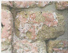
Stone Wall of Oglethorpe Lane Building
