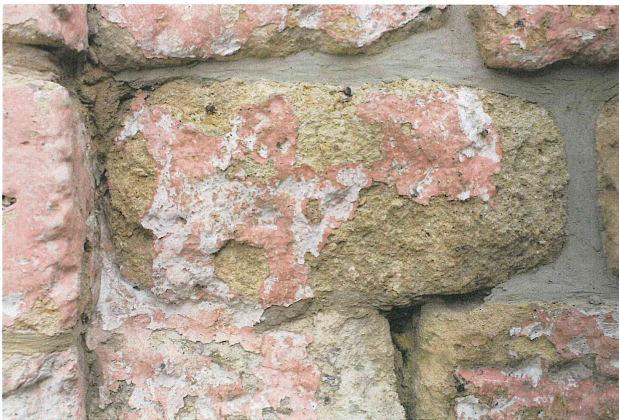
Stone Wall of Oglethorpe Lane Building
