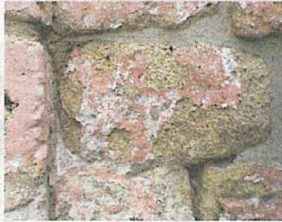
Stone Wall of Oglethorpe Lane Building
