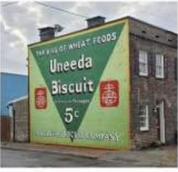
FULL RESTORE -NEW 1897 BILLBOARD RESTORATION
