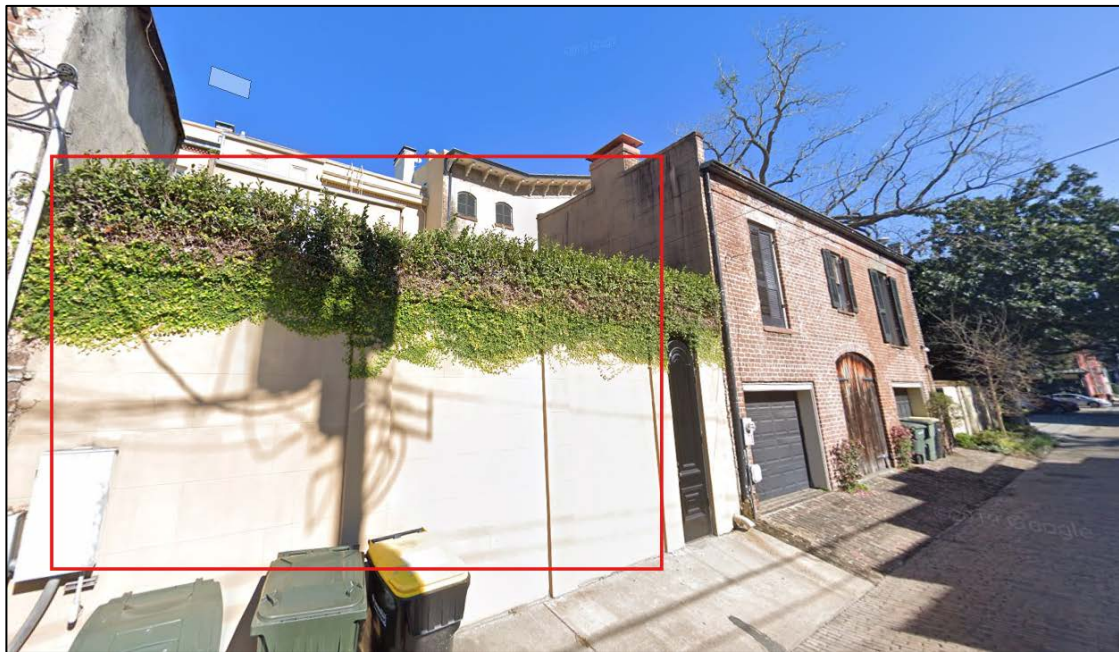
Accessory Structure to the East of the Parcel
