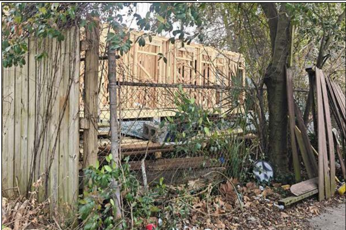
Photos of the Structure from Site Visit on February 11, 2026
