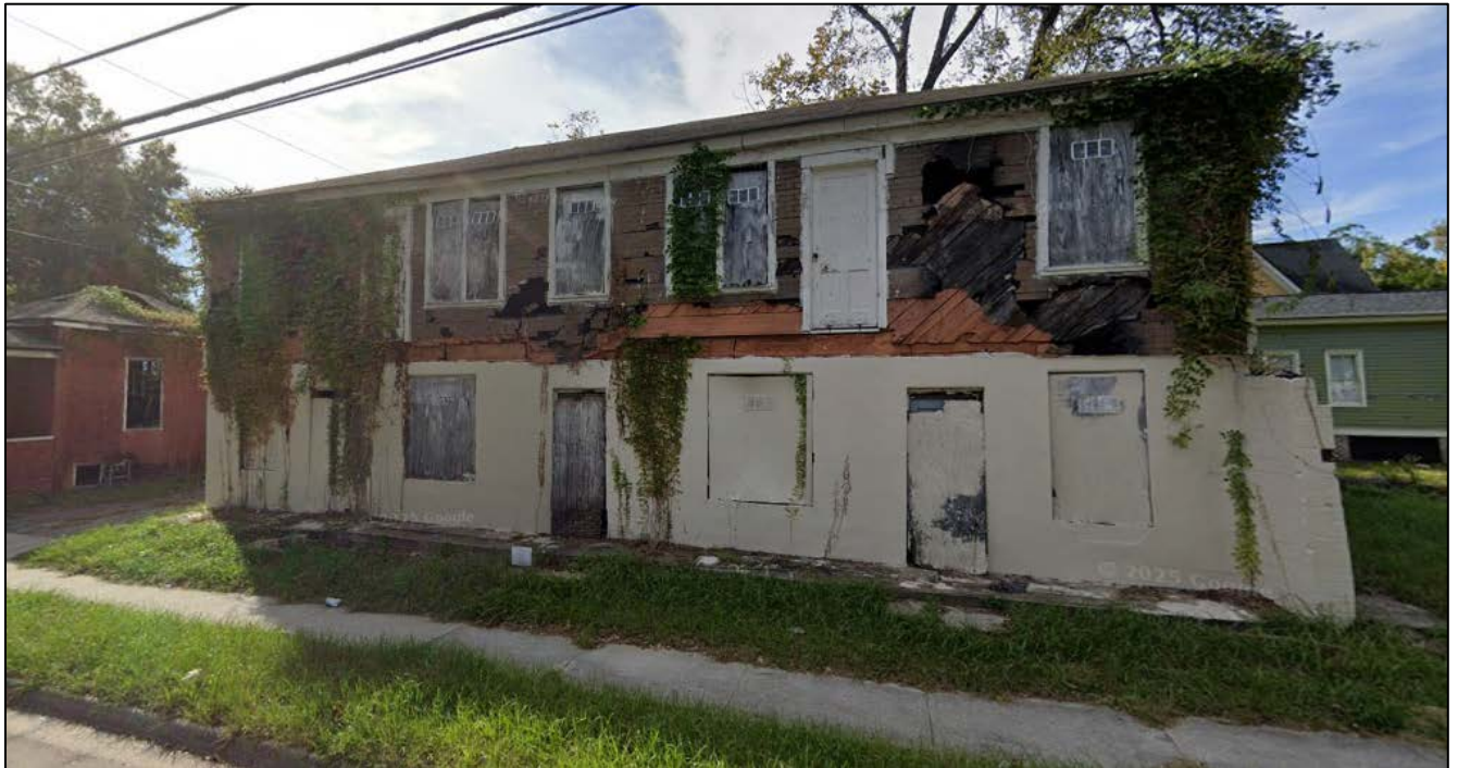
View from Side of Property on Burroughs St (Google Street View, Oct 2025)
