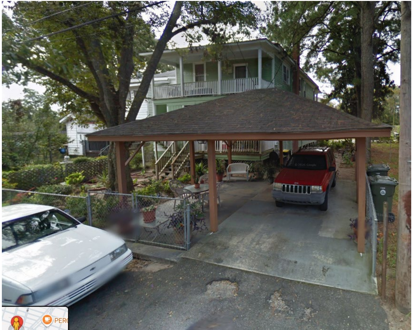
Street view from 2014 showing the previous carport
