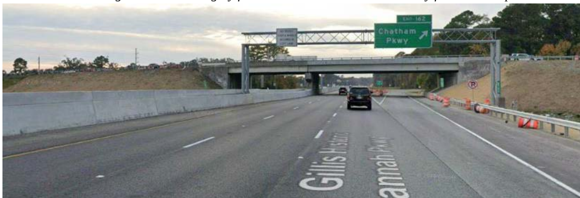
Google Streetview imagery from November 2025 shows visibility from westbound I-16
