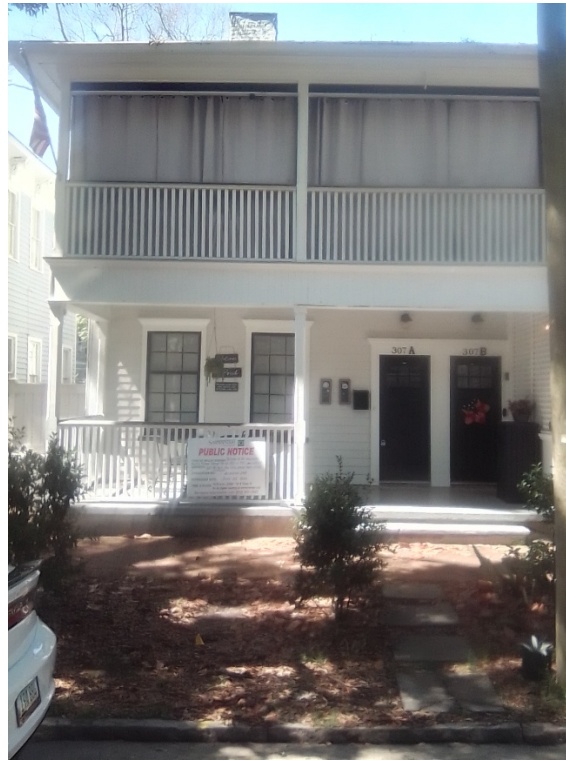
Front View of 307 W. Park Avenue
