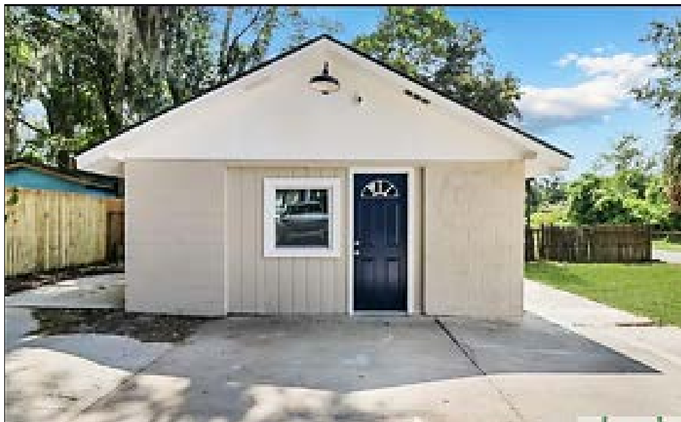
Existing ADU Photo #1 located at 3032 Grenoble Street
