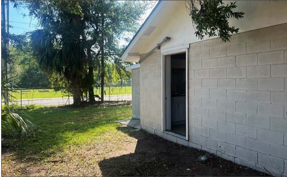
Existing ADU Photo #2 located at 3032 Grenoble Street
